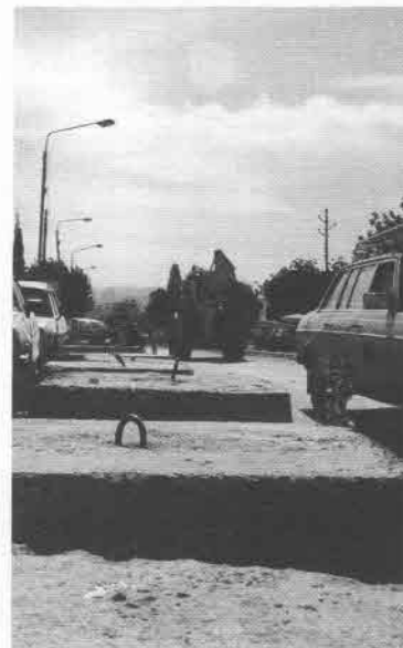
Bulldozers and barricades prevail in Bethlehem as construction continues.
